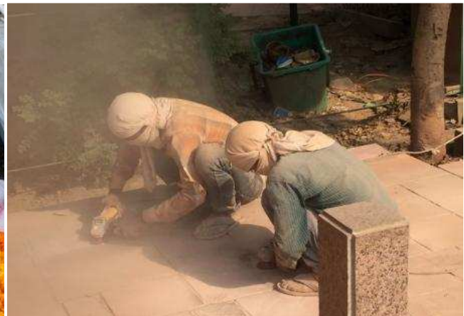
Posure to silica is a common occupational are informal workers health hazard
