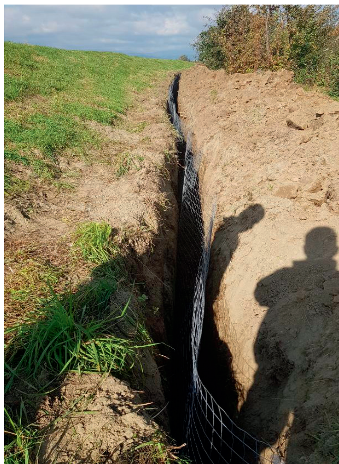
Fig. 3. Inserting the mesh into the ditch
