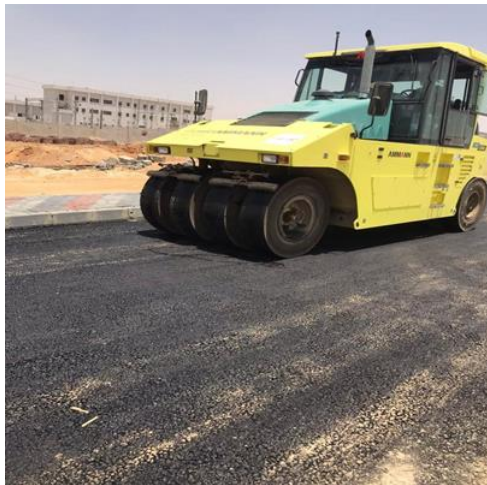
Figure 6: Pavement Condition in Libya.
