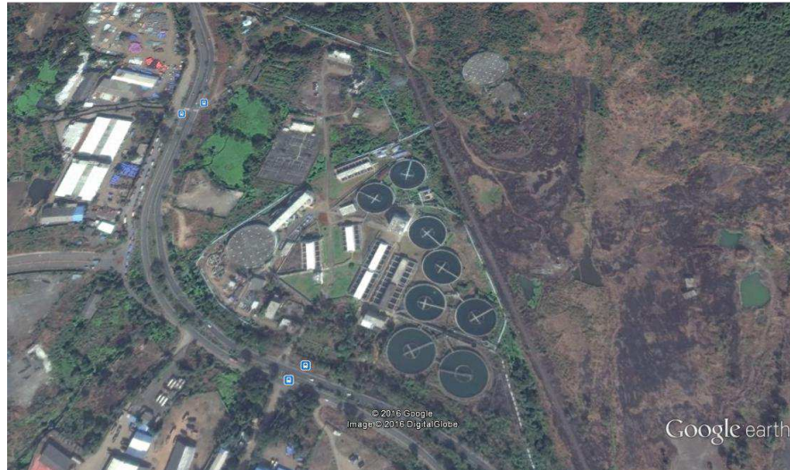
Figure 1: Google Image of Water Treatment Plant
