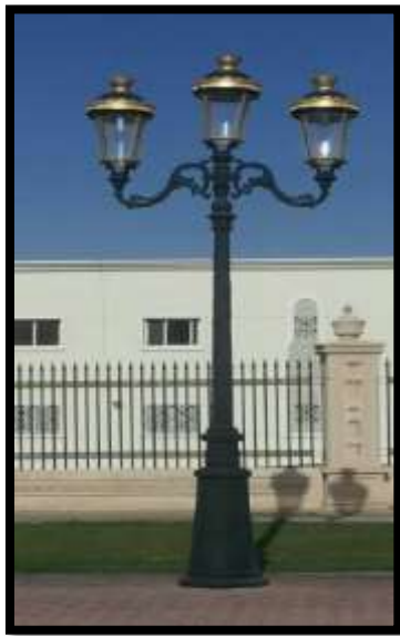
Fig-1: conventional Street Lamps in AUS
