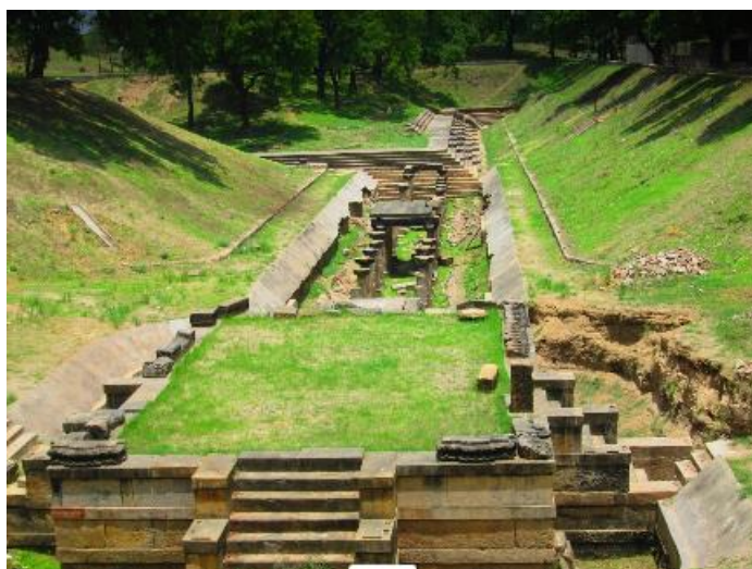
Photo 2: Sahastralinga Tank Platform
