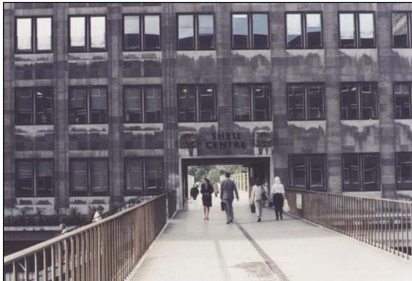
Fig. 4 – The Shell Centre: Note the distinctive black and white appearance of Portland Stone (Source: author).
