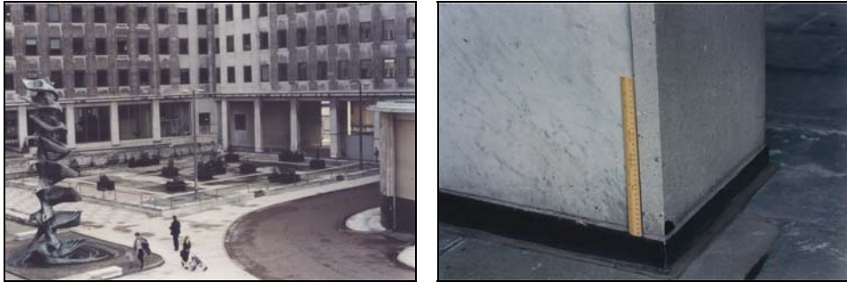
Fig. 5 – (Left) The Shell Centre: Courtyard of U-shaped block; (Right) Detail of low part of columns surrounding the courtyard; scale bar is 30cm in length (Source: author).
