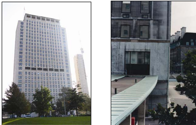
Fig. 3 – (Left) The Shell Centre: South Bank (Source: William Bondin); (Right) In the multi-storey building of the Shell Centre, Portland stone and marble are used to clad the upper and lower storeys respectively (Source: author).
